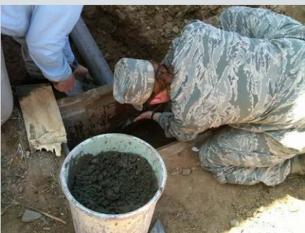
Capt Tracy Brannock, USAF, Cementing Sewage Piping
