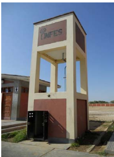
Manuel Pio Water Tank and Cistern
