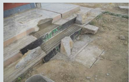
Fresh Cement After Connecting the Pipes
