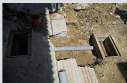
Sewage Piping Construction
